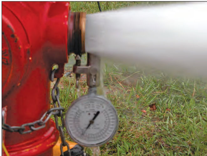
Figure S8.9. Flowing hydrant with standard pitot gauge attached to hydrant used to conduct fire-flow test (gauge reads pressure and flow), Hadnot Point–Holcomb Boulevard study area, U.S. Marine Corps Base Camp Lejeune, North Carolina, August 25–27, 2004.
